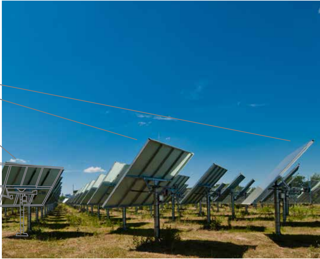
The heliostat field around the central tower receiver at KAM's demonstration plant in Jülich, near Cologne, Germany
